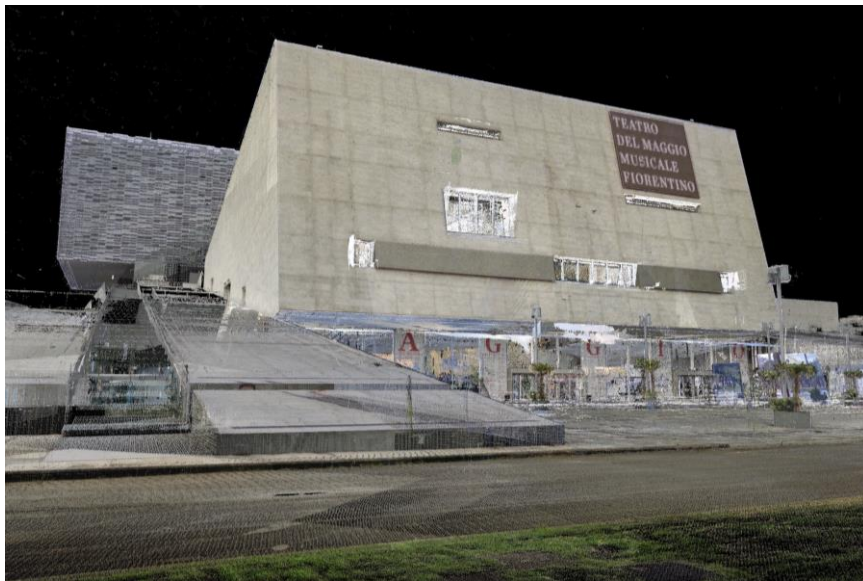
Coloured point cloud of the external areas of the Opera di Firenze
