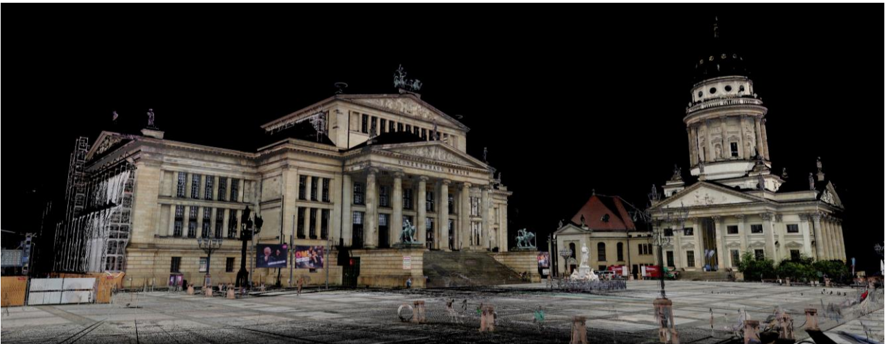
Coloured point cloud of the external areas of the Konzerthaus Berlin and Gendarmenmarkt Square
