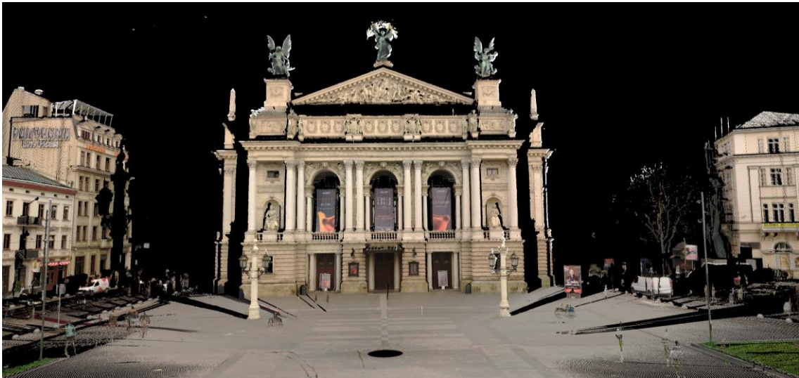
Coloured point cloud of the exterior of the Lviv Opera House acquired and processed by the UNIFI-DIDA team
